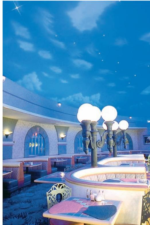
**Plate 6-2 (left)** Layers used to make artificial sky and day/night effect. Deep blue uplight, dimmed incandescent globe lights and sconces, and white fiber-optic star field. Programmed cross-fade dimming creates realistic day/night transitions. *Photo: J. Benya*
